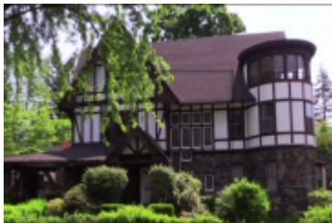
Yonkers to see its first mosque, despite controversy
